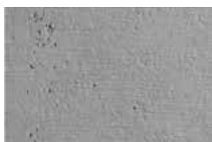
Coarse concrete technique
