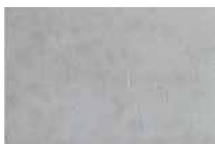
Smooth concrete technique
