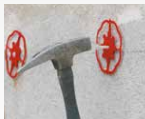
The Baunit adhesive anchors are inserted into the borehole and secured with plastic nails.
